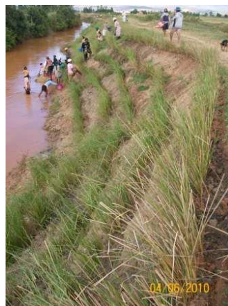
The maintenance work was here very important, because of the long period without rain (8 months), pressure from cattle and fire. The hedges had to be enough strong when the rainy season will be start with big flow of water!
