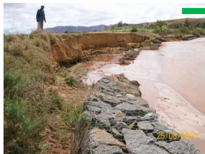
The maintenance work was here very important, because of the long period without rain (8 months), pressure from cattle and fire. The hedges had to be enough strong when the rainy season will be start with big flow of water!
